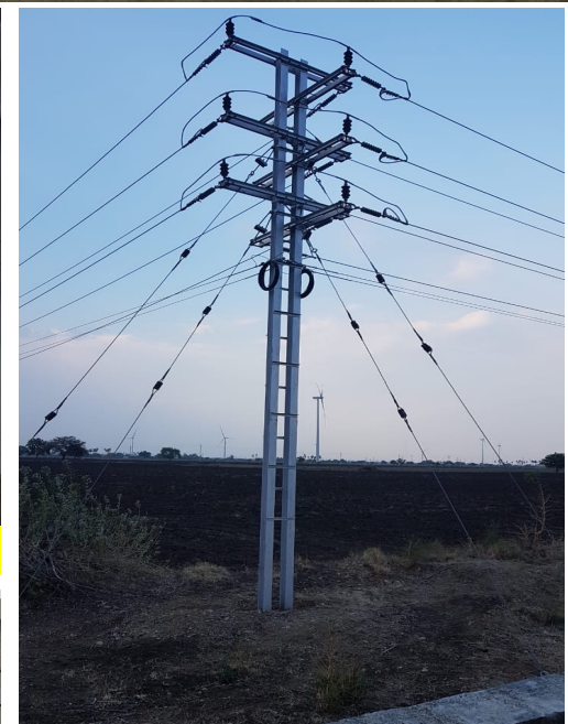
33KV DC line with Panther conductor on RSJ poles for 25Km @ kayathar
