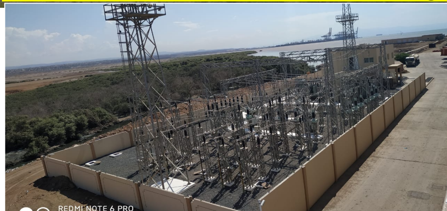
63KV /20 KV, 25MVA GIS Hybrid station at East Africa
